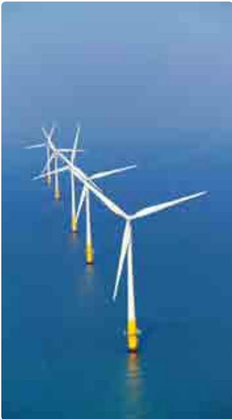
Offshore Wind Farm
